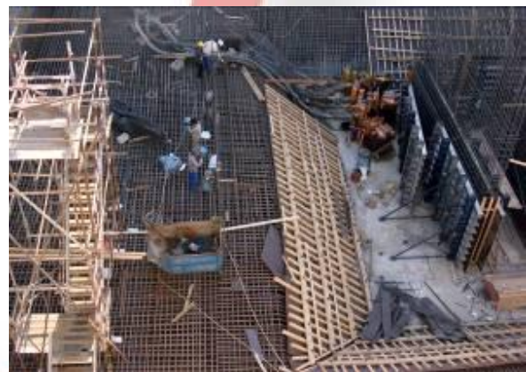
Shuttering of wind Tower I
