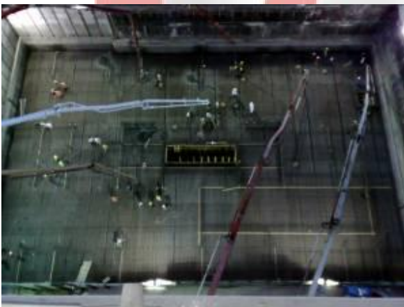
Concrete pouring of Wind Tower II
