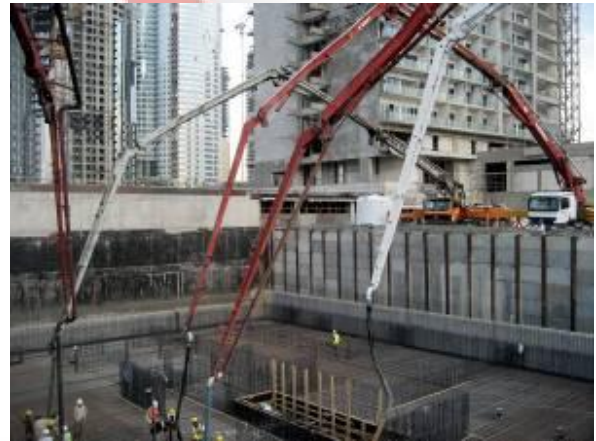
Concrete pouring in Wind Tower II
