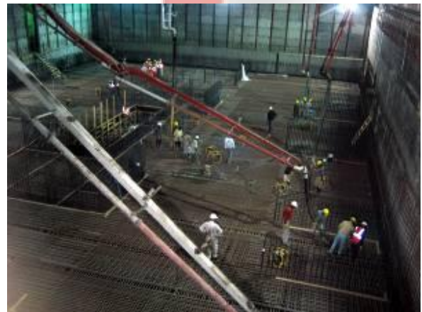
Concrete pouring in Wind Tower II (night shift)
