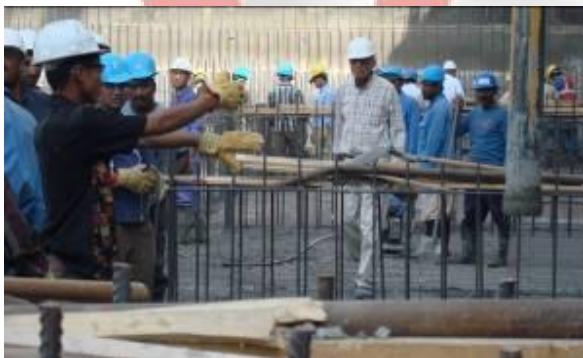
Concrete pouring in Wind Tower II
