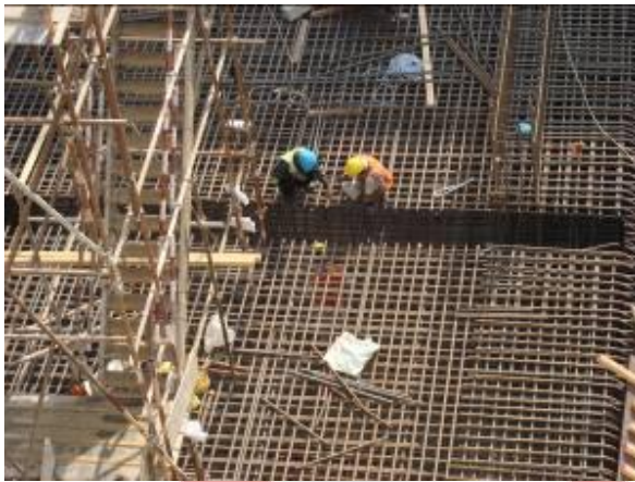
End of shuttering of Wind Tower I
