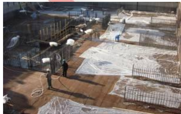
Stage of curing in Wind Tower II
