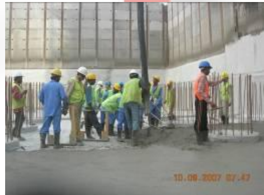
Horizontal Water Proofing Wind Tower II
