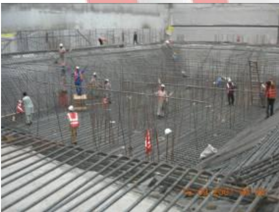
Reinforcement Wind Tower I
