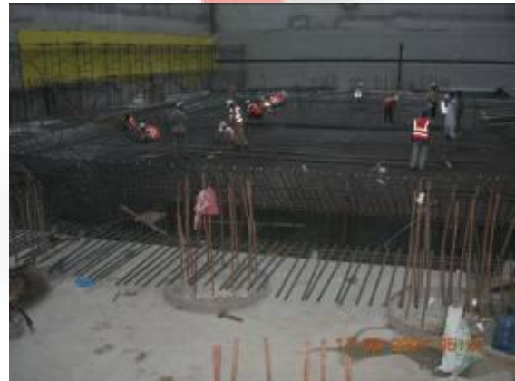
Reinforcement Wind Tower I
