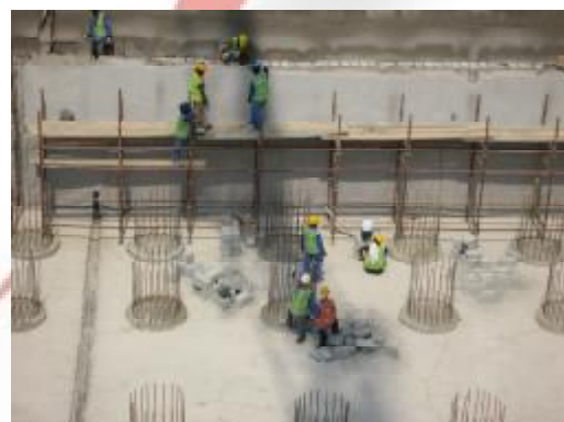
Vertical Water Proofing Wind Tower II
