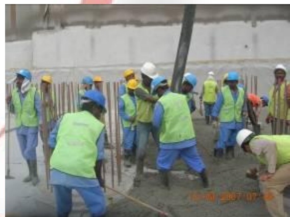
Horizontal Water Proofing Wind Tower II
