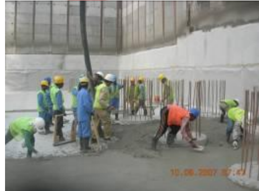
Horizontal Water Proofing Wind Tower II
