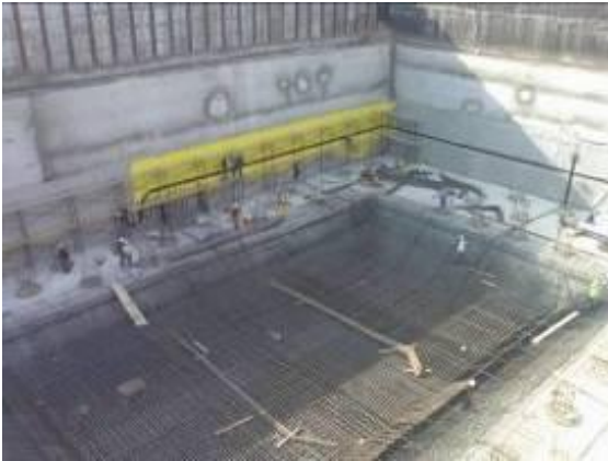
Reinforcement Wind Tower I
