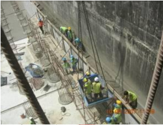
Vertical Water Proofing Wind Tower II
