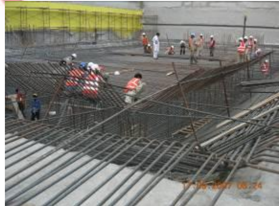
Reinforcement Wind Tower I
