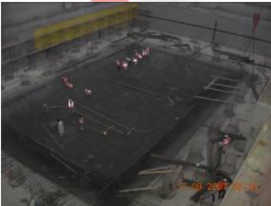
Reinforcement Wind Tower I
