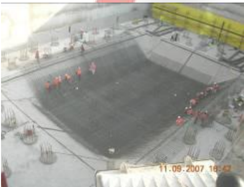
Reinforcement Wind Tower I
