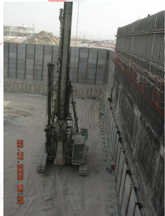
Drilling Machinery at Wind Tower II's Construction Site
