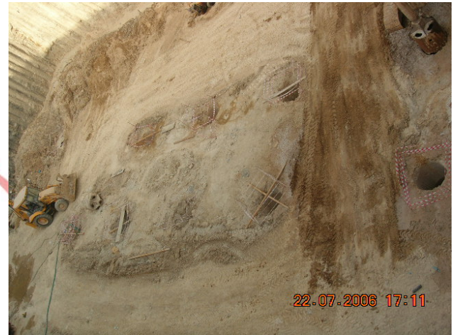
Drilling for Wind Tower I
