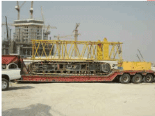
Tower Crane Delivery
