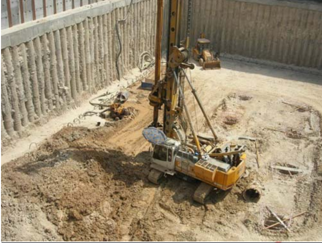
Drilling for Structure at Wind Tower I
