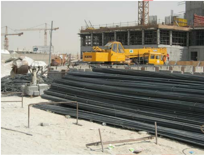
Steel bars delivered for substructure
