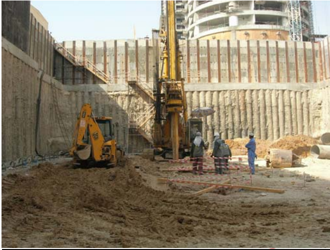
Drilling for substructure of Wind Tower I
