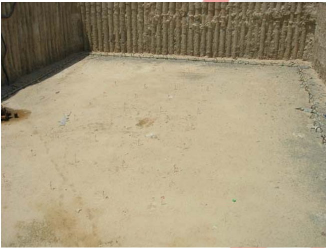
Demarcation for Piling
