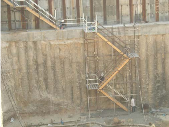
Staircase Installation in Wind Tower I Construction Site
