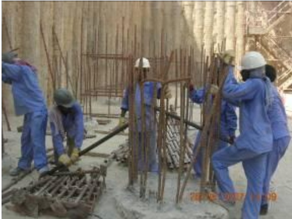
Installation of Scaffolding Wind Tower I
