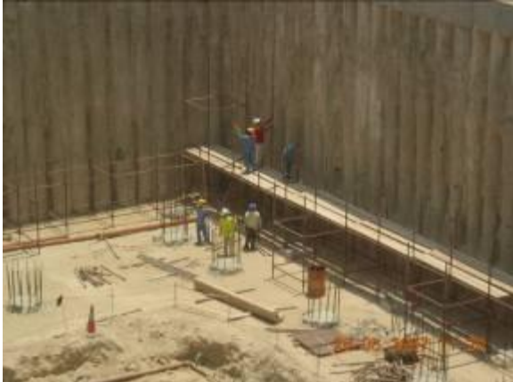
Installation of Scaffolding Wind Tower I
