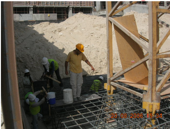
Tower Crane Reinforcement for Wind Tower II
