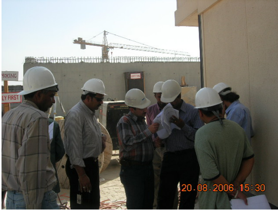
Pile Checking for Casting for Wind Tower I
